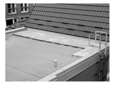
3. Some of the well-crafted flashings around the nave stained glass windows. Here the new waterproof membrane is below both the insulation and a concrete surface to protect it from falling ice and prevent the kind of build up that has necessitated shoveling this roof in the past.
